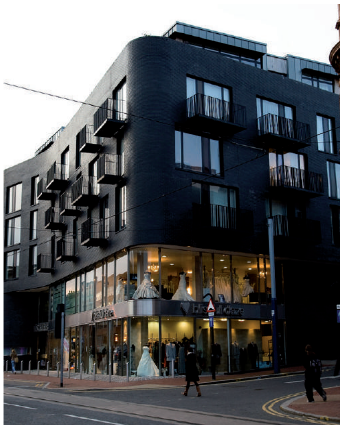
Figure 9.4: Active frontages at Accordia, Cambridge (David Millington Photography Ltd)
