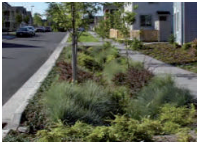
Figure 13.5: Vegetated drainage channel
