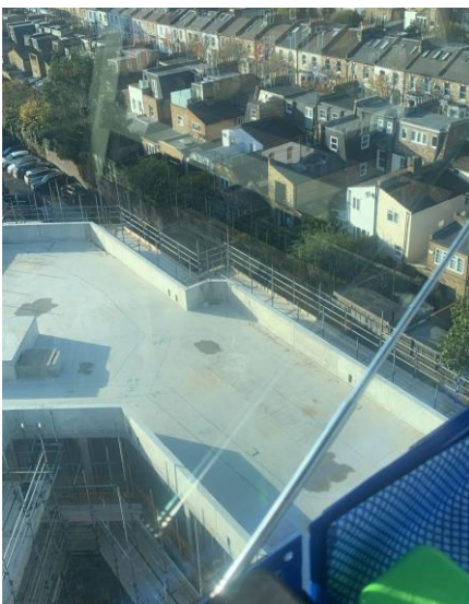
View of Block C roof
