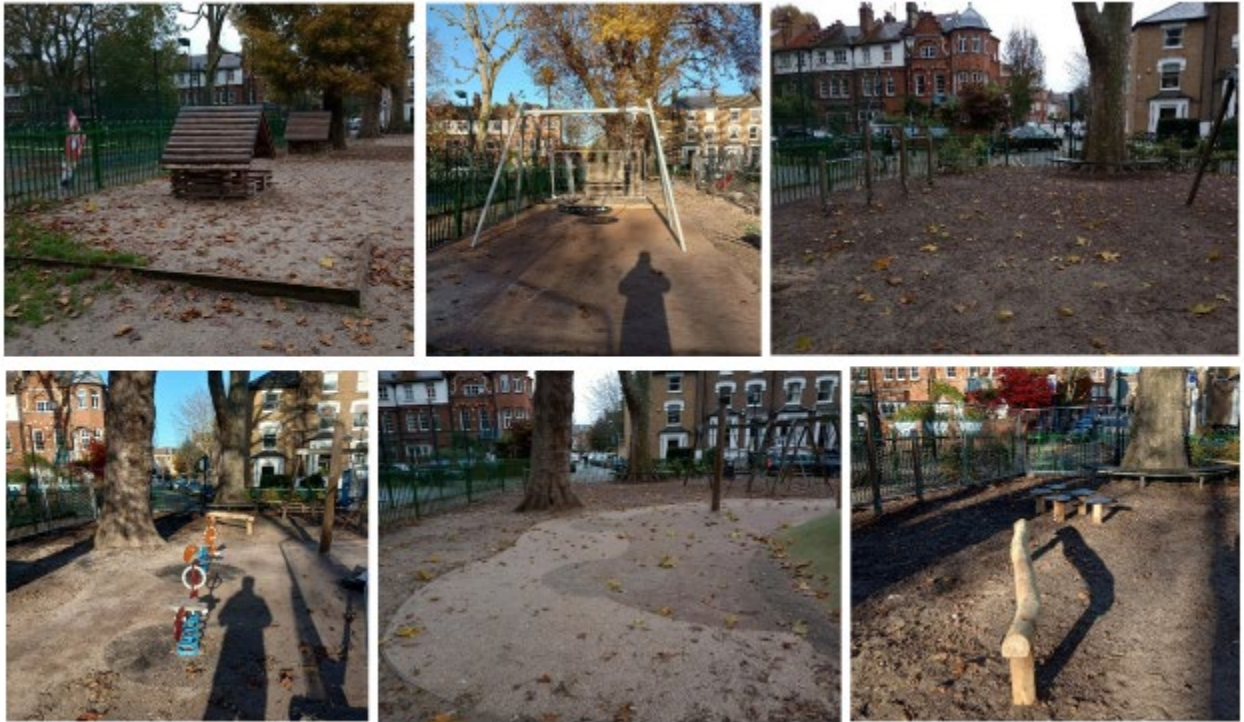
Figure 20: Brook Green Playground - Upgrade of the playground installing 13 pieces of new play equipment including, swings, play panels, springers and activity trail.
