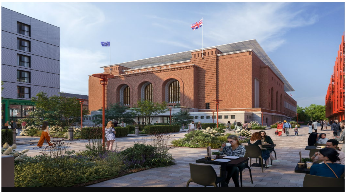
Figure 7: Exterior Town Hall, Civic Campus
