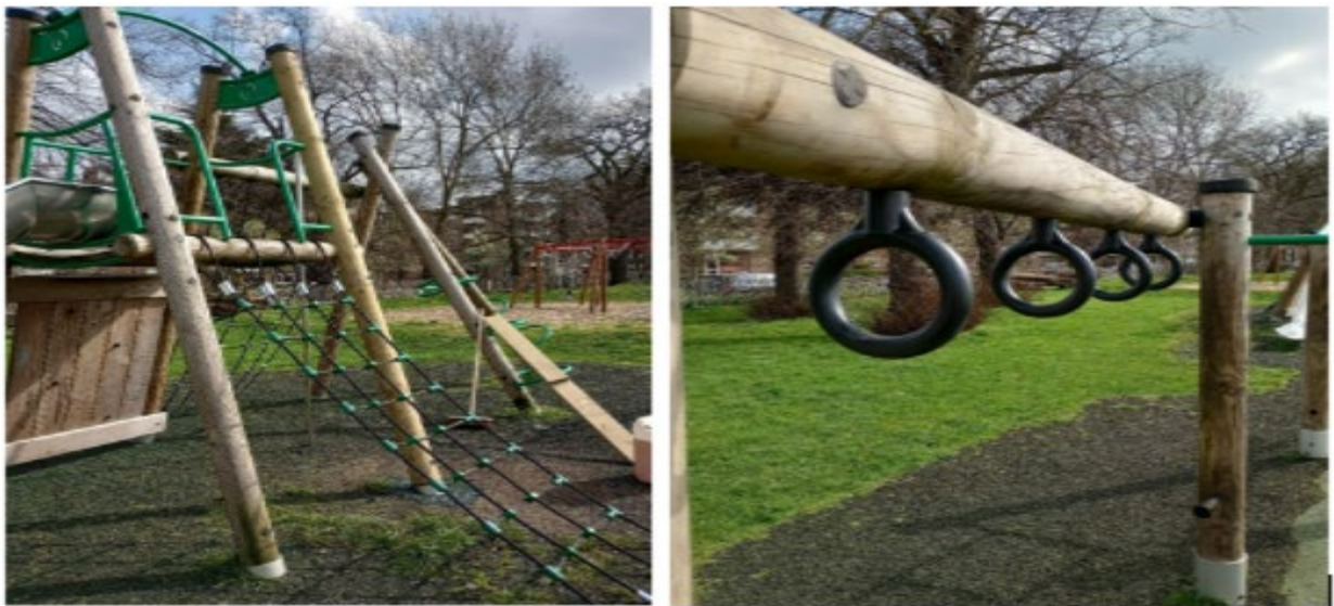
Figure 21: Hurlingham Park - Repairs to multi-play unit, eradicating issues from annual inspection reports. New ropes, and posts.
