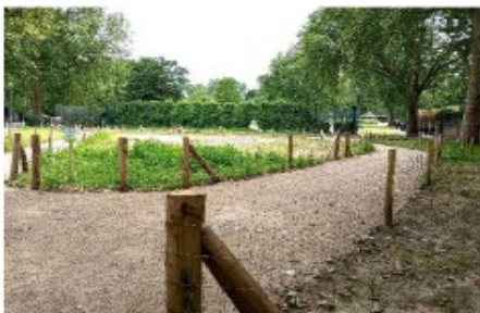
Figure 25: Eelbrook Common - De-paving project 2,500 m 2 of tarmac and concrete surfacing was dug out and replaced with permeable gravel pathways and planting. The area had previously been a concrete paddling pool.
