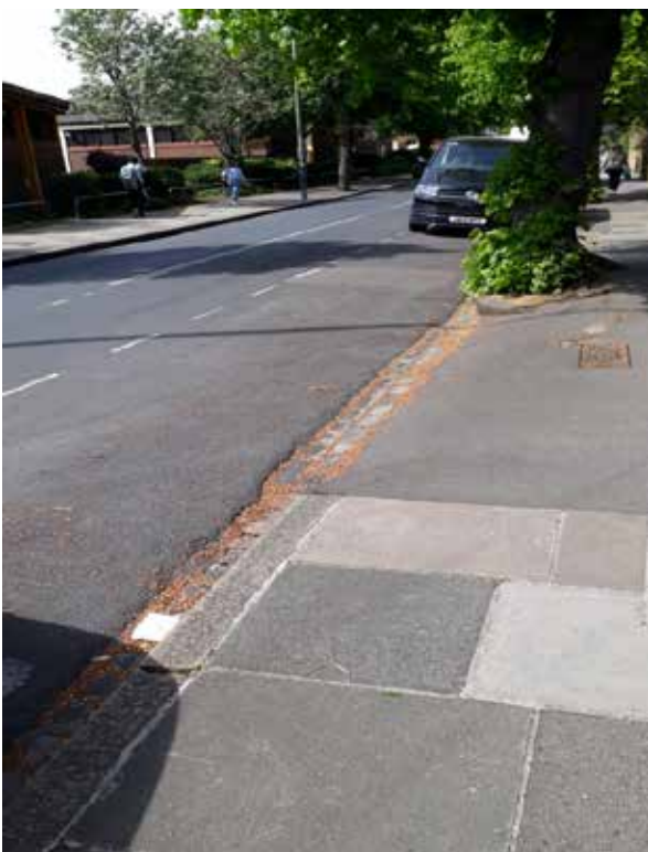
[Continuous parking bay in front of dropped kerb]
