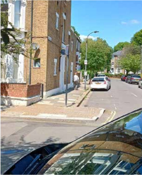
[Lena Gardens – misaligned no through road sign] [NB no keep right sign on build out here]
