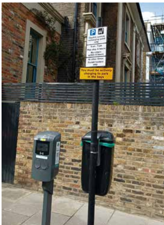
[Could the sign and charge point be combined and be designed in some cleverer way?]
