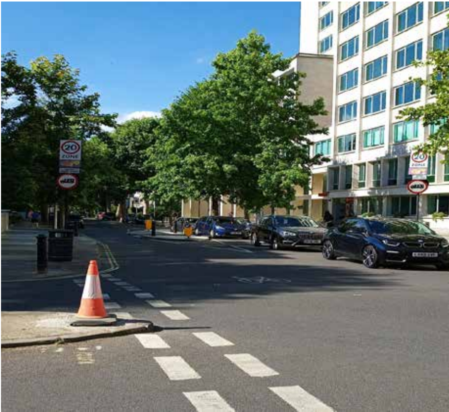
[20 MPH signs in a 20 MPH zone/Grove Home zone signs/ on both sides of carriageway, partly obscured by trees. HGV Ban sign obscured/not obvious] [NB missing bollard on traffic island]
