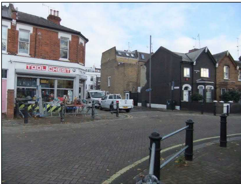
Figure 65: Image of Existing Junction at Iffley Road (Tool Chest) showing 'dog leg' and Van Parking Obstructing View
