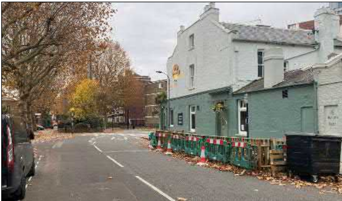
Figure 25: Photo of Dalling Road (Thatched House) Before
