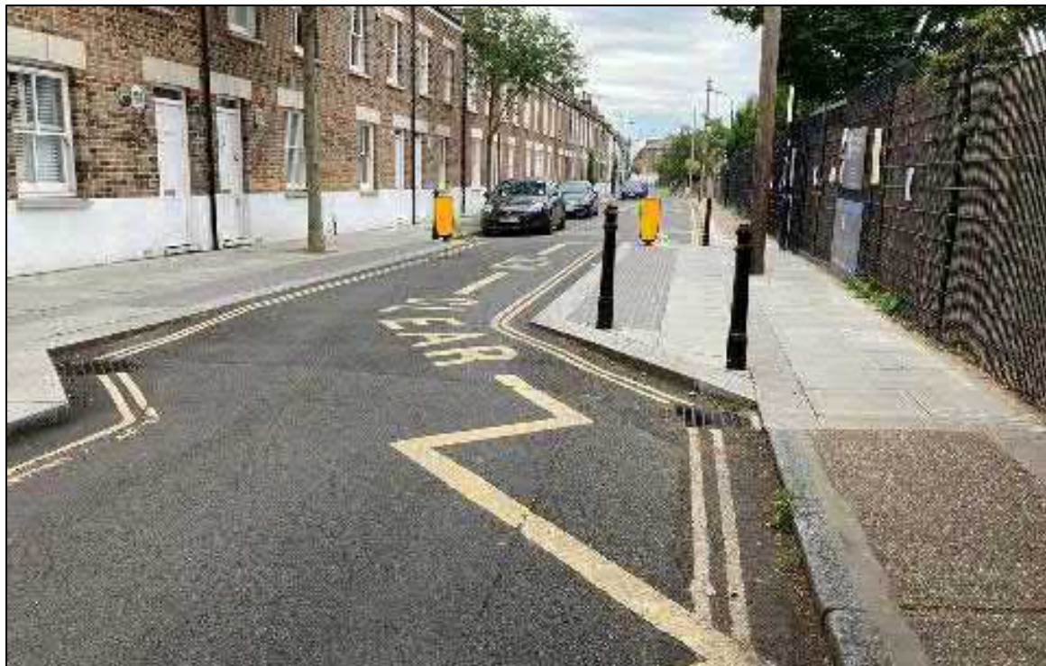
Figure 70: Image of Existing Arrangement on Banim Street
