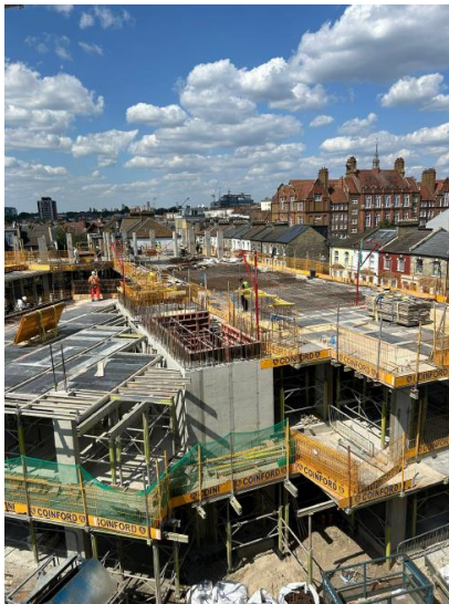
Left: Aerial view from tower crane overlooking Block C
