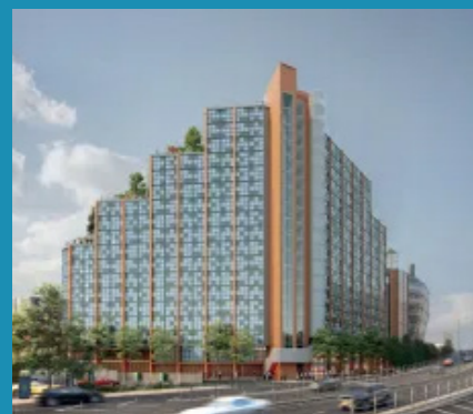
161 Talgarth Road - Under Construction
