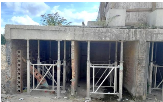
Completed support works to the pedestrian walkway
