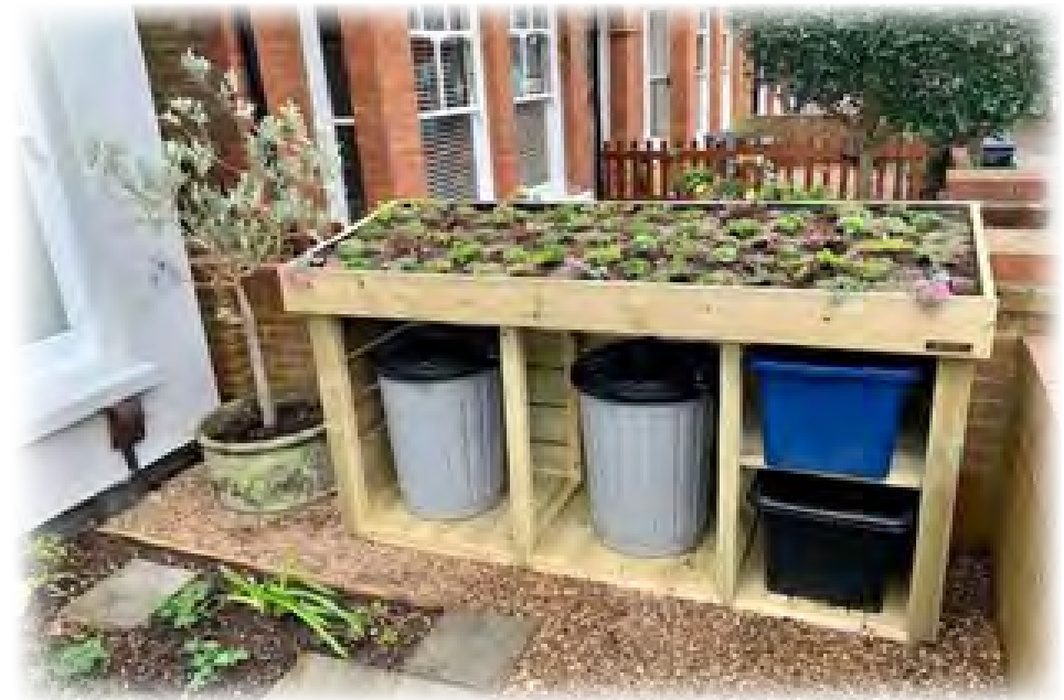
Image 17: Waste Storage with a green roof
