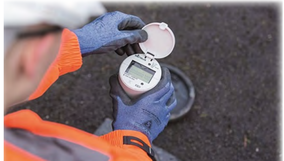
Image 4: Fitting a water meter
